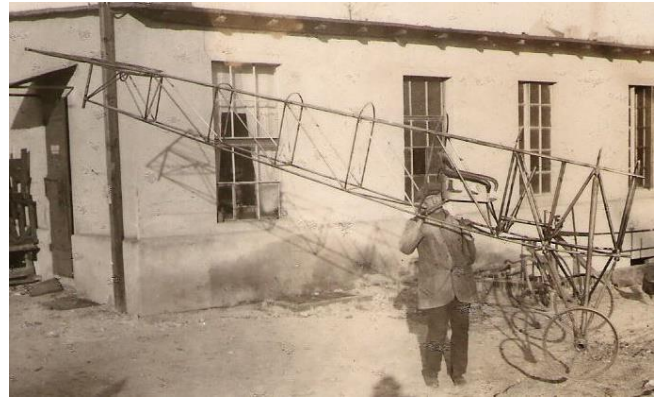
(a) Light-weight steel tube frame
