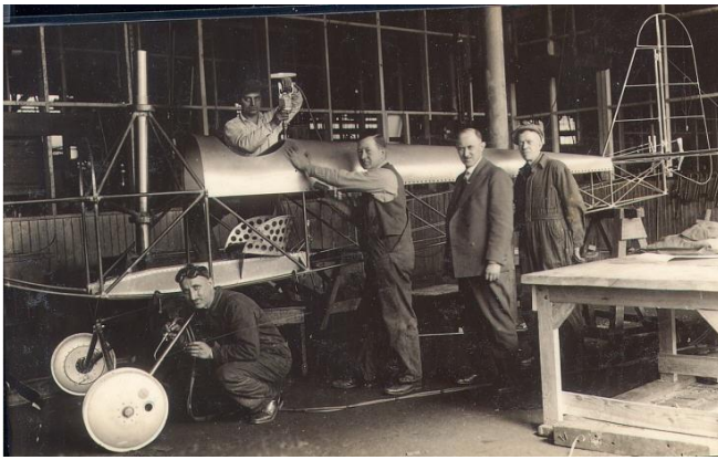
(a) Fuselage frame assembly
